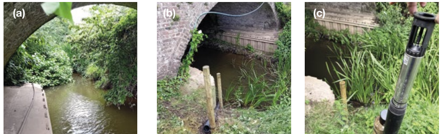
Water-level sensor installed in Strine catchment in 2024. (a) suitable site identified with access and unobstructed water flow, (b) trenching for sensor pipework (c) wireless sensor installed within access pipe.
